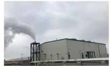
Hanford Site WTP Steam Plant
